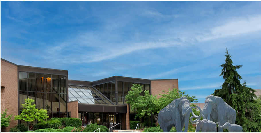
Future location of Cincinnati Museum Center's treasures and research facility.
